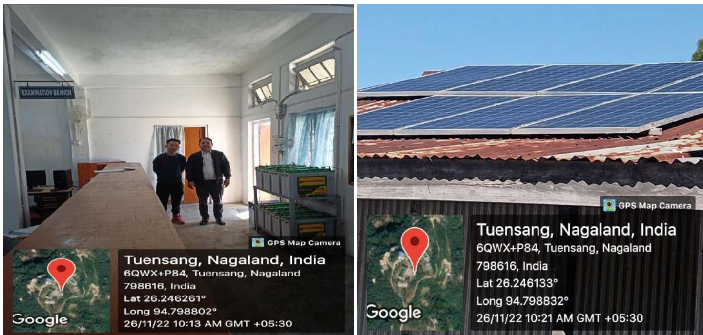
Installation of 3KVA Solar power
