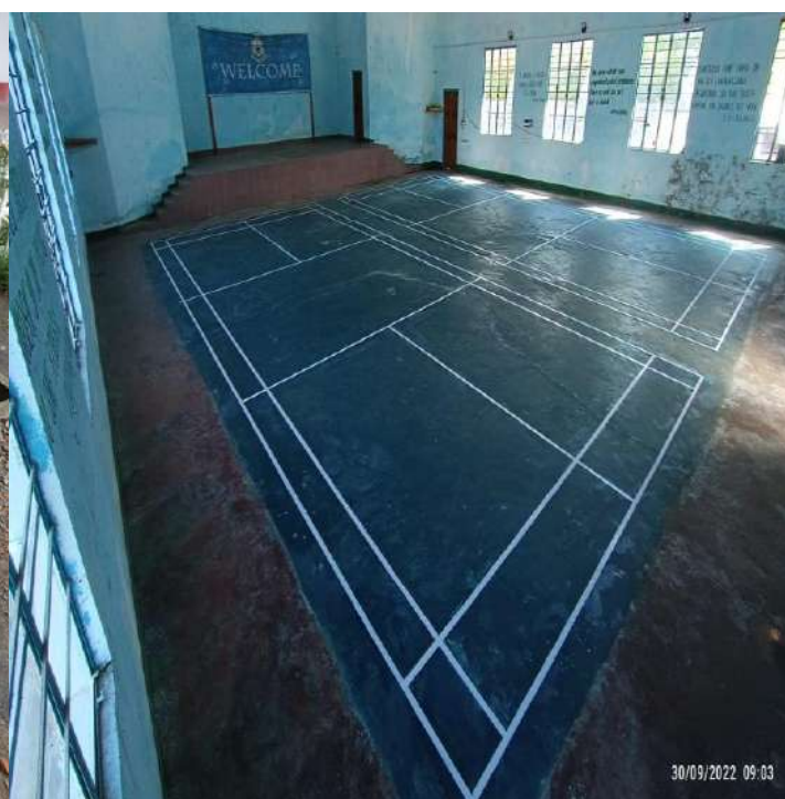
Multipurpose Hall concrete flooring and permanent laying of badminton court (2 nos)
