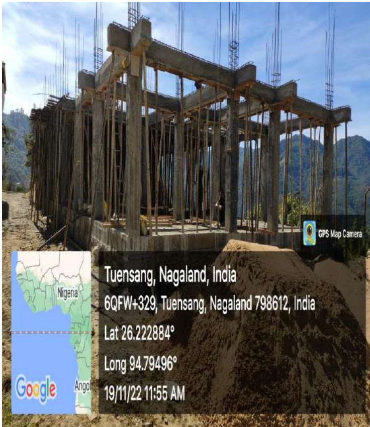
Newly construction: Extension of Classroom
