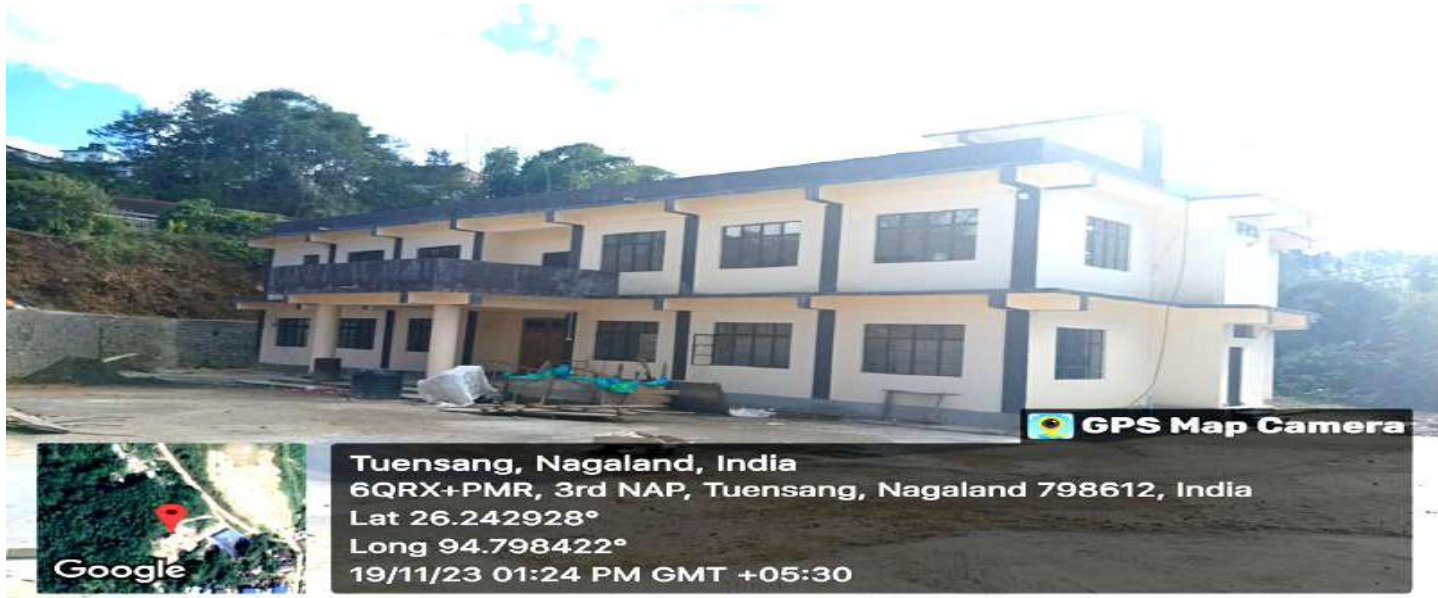
Under Construction: Girls Hostel
