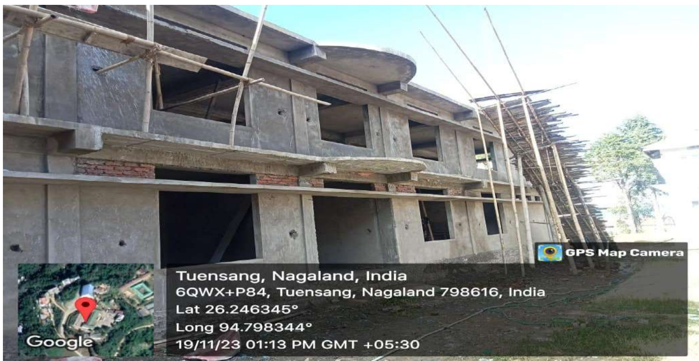
Under construction : Extension of Classroom
