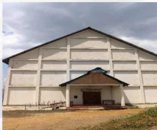
SCC MULTIPURPOSE HALL
